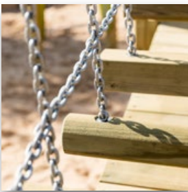
Suspension bridge: Softwood Chains: Steel galvanised
